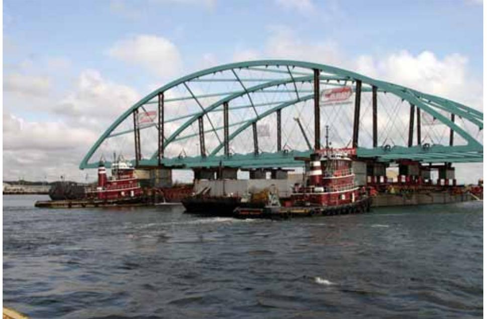
Mammoet had turned the two barges into a giant catamaran, holding them in position with two 100-foot sections of crane booms and steel cables. The bridge was loaded across the two barges, with its ends overhanging on each side. "I don't think that's been done very often, if ever," said Richard Zondag, Mammoet's operations manager.
