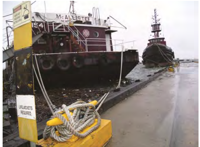
The MCALLISTER 154 and the COLLEEN MCALLISTER on Tuesday after the storm, as the water receded.
