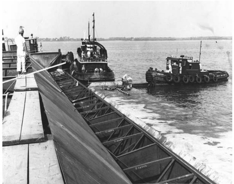
Towing and positioning tunnels in the Chesapeake.
